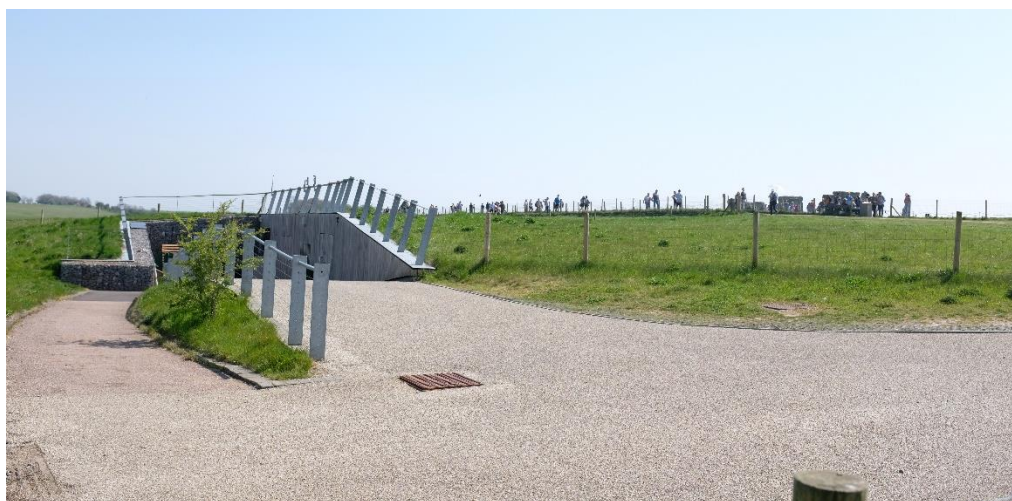
Figure 6 Fencing around former Visitor Centre and swathe of tarmac visible from Stonehenge Monument field, April 2019
